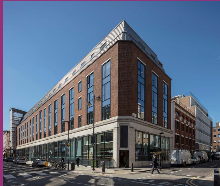
The Johnson Building
